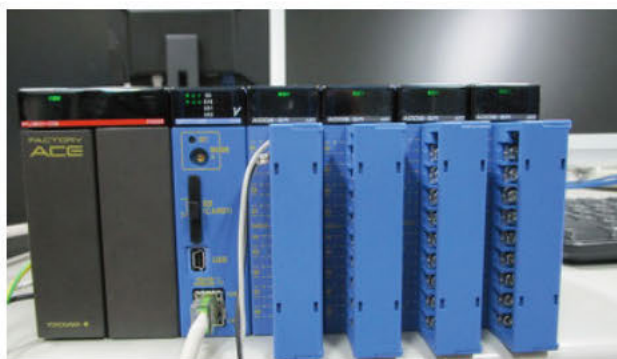
Programmable Logic Controller (PLC: YOKOGAWA)
