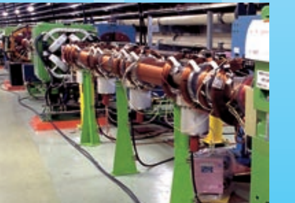
Solenoid magnets for positron ring: Solenoid magnets are installed over the entire positron ring to suppress the harmful build-up of electron clouds. KEKB showed a dramatic increase in luminosity after their installation.
