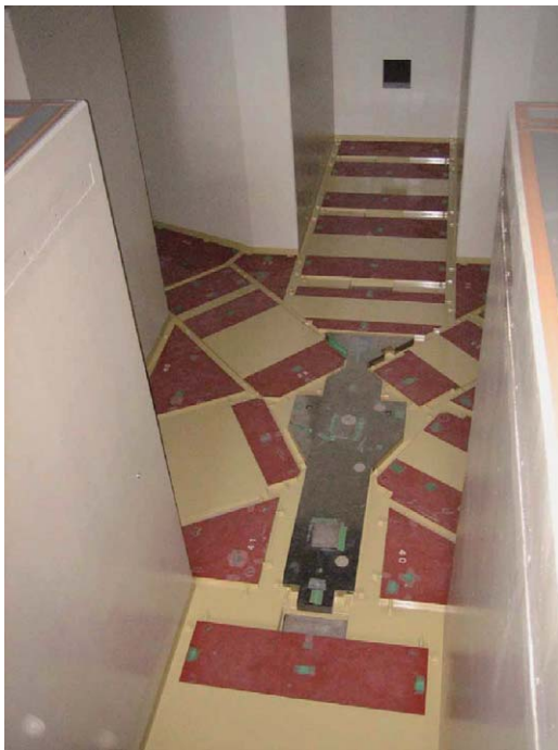
Fig. 3. View of the alignment plates installed in the M2 tunnel around the muon target area.
