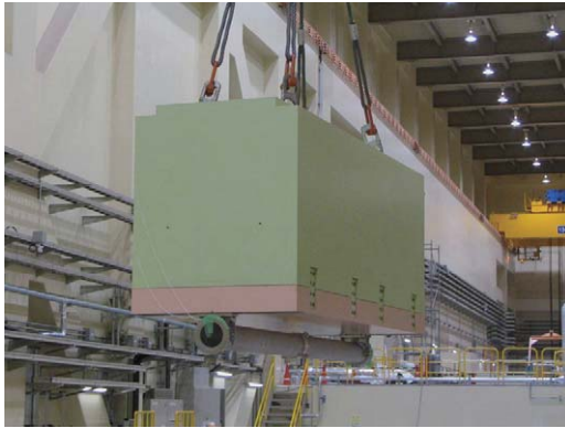
Fig. 5. Beam duct assembly for the M2 primary proton beamline.
