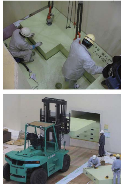
Fig. 6. Installation of the temporary concrete blocks in the exit of the secondary muon channel (H-line) that will not be operational on day one: with a crane inside the M2 tunnel (above) and with a forklift from the experimental hall (below).
