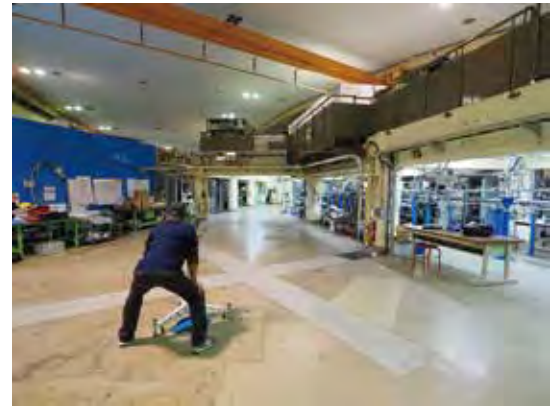
Survey of the proposed site for the construction of the R&D beamline (August 2023). The removal of the former BL-11A, B, and D has been completed and some of the equipment will be moved to newly constructed BL-12A.
