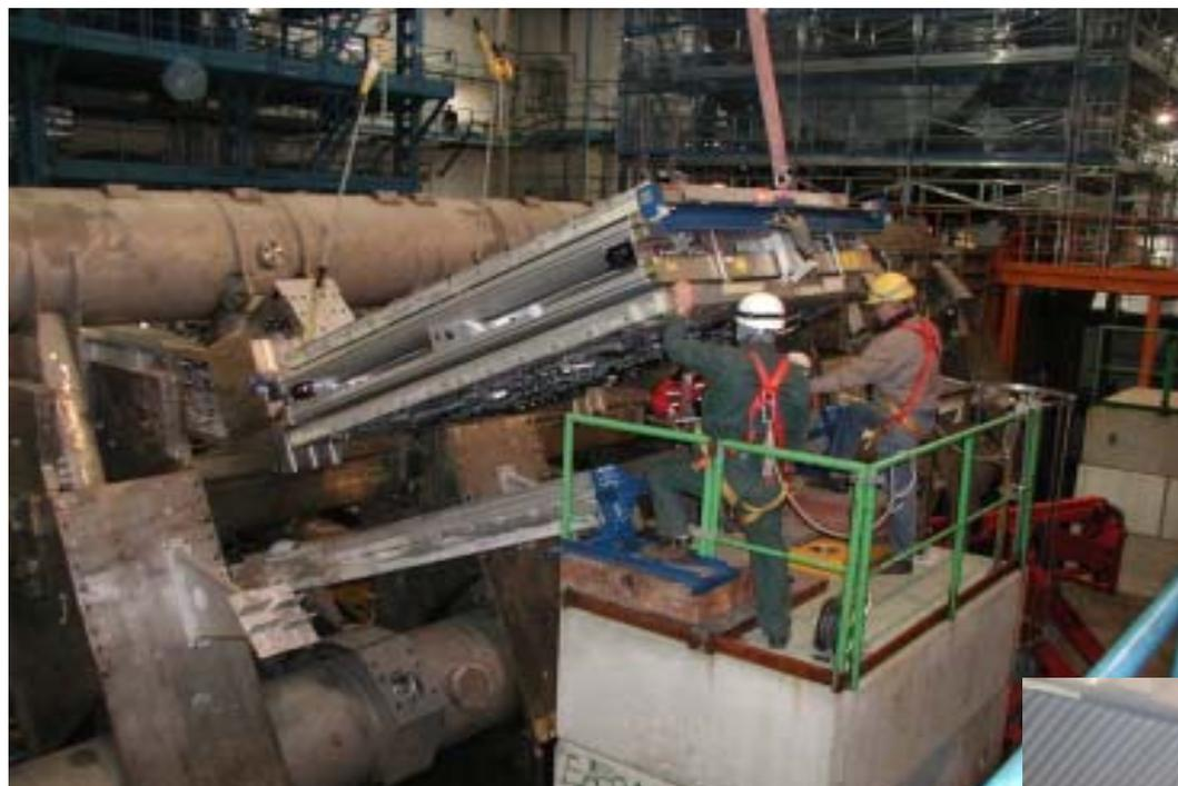
The installation of the barrel muon station has started in the feet region of the detector
