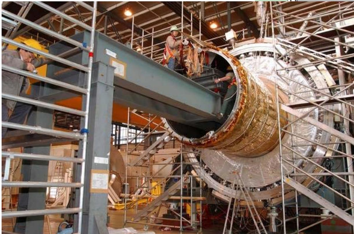
The solenoid has been inserted into the LAr cryostat at the end of February 2004, and it was tested at full current (8 kA) during July 2004
