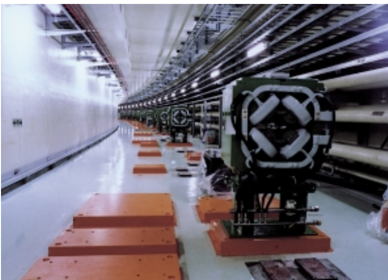
Quadrupole magnets for LER placed in the TRISTAN tunnel
