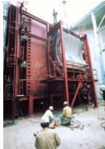
installation of near-detector in progress
