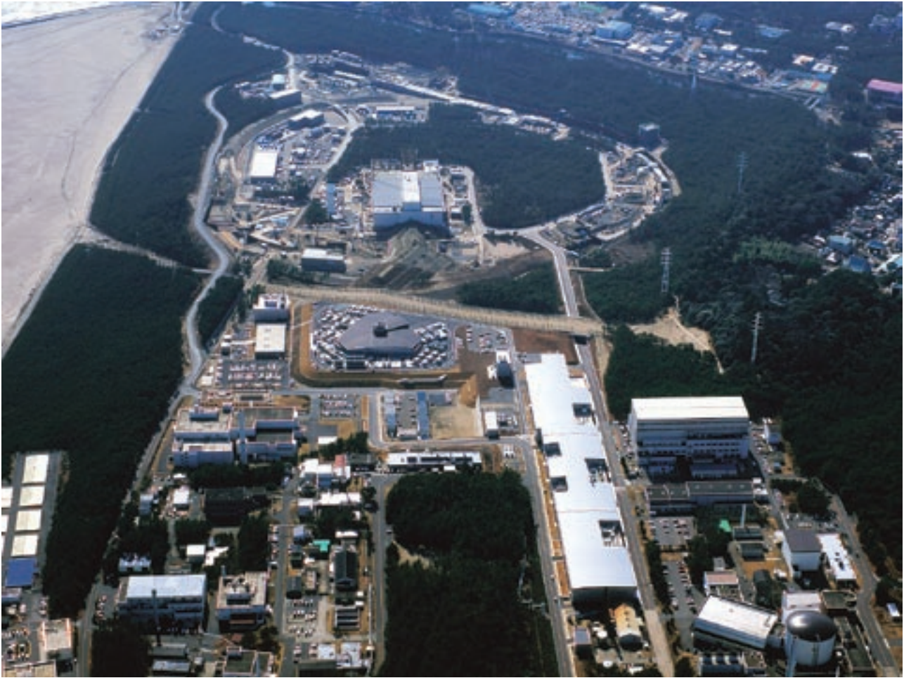
An overall construction status of the J-PARC, as viewed from the sky. The photo was taken on February, 2006.
