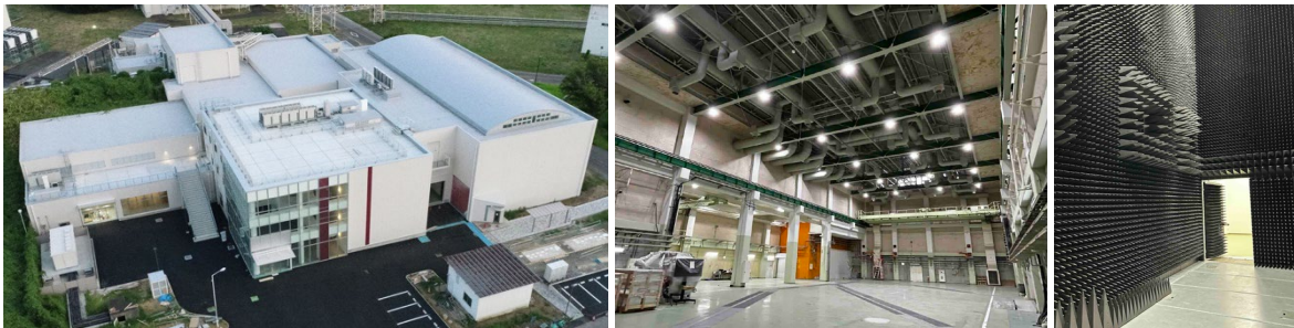
Figure 16 QUP building complex, the experimental hall area, and anechoic chamber.
